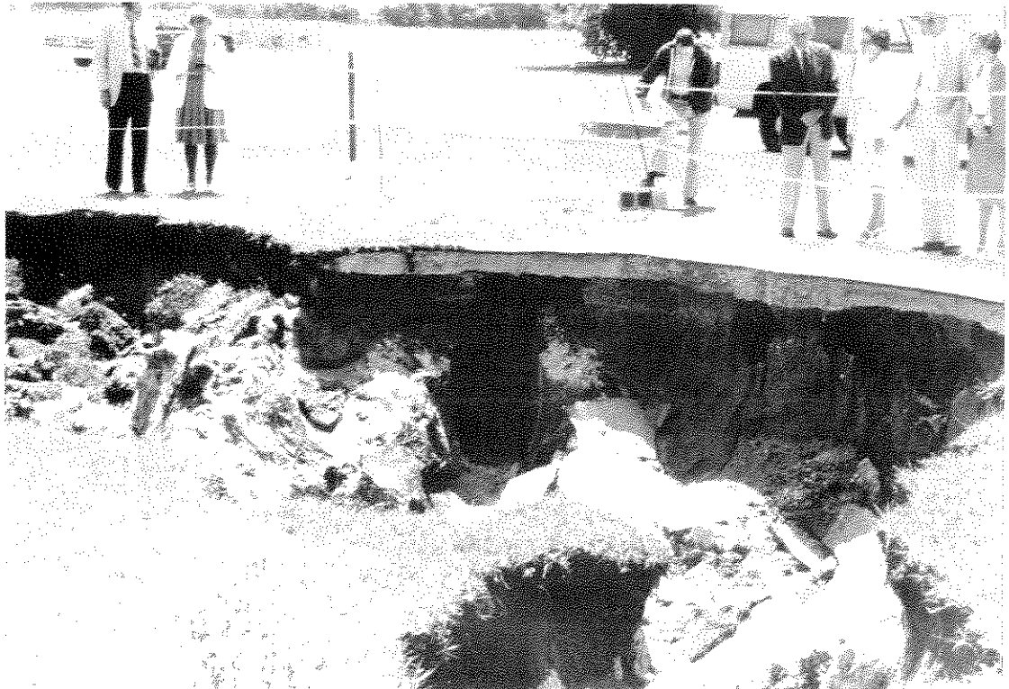
Figure 26. Sinkhole in City of Ocala formed during the flood of April 1982. Florida Geological Survey photograph.
