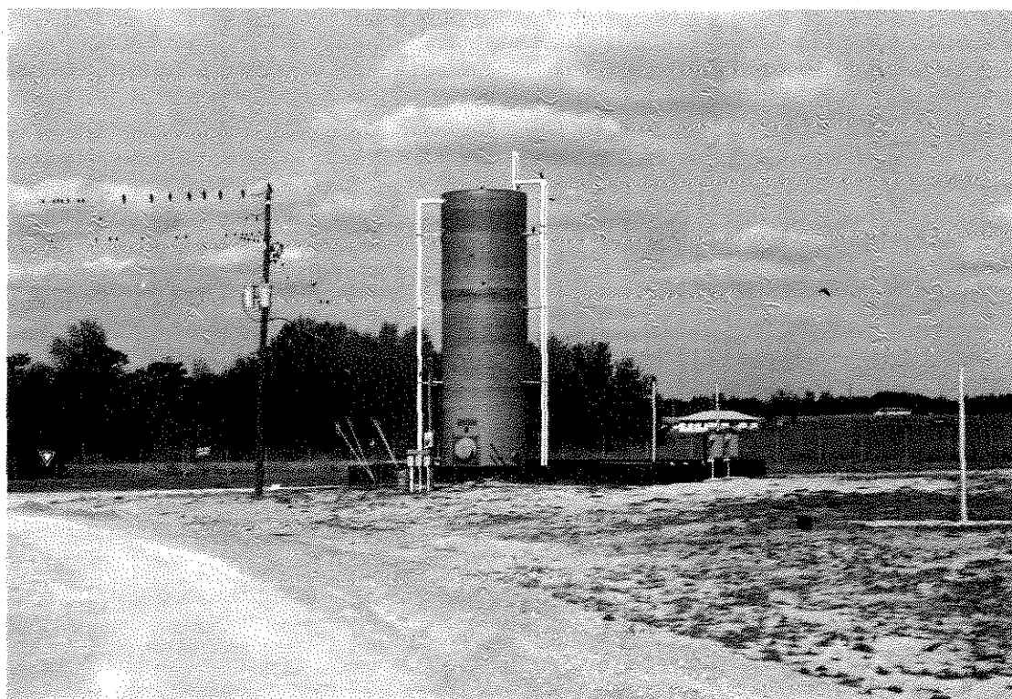
Figure 47. The 30,000 gallon leachate holding tank at the Marion County landfill, showing some of the pipes that connect to those shown in Figure 46. Florida Geological Survey photograph, February 1989.
