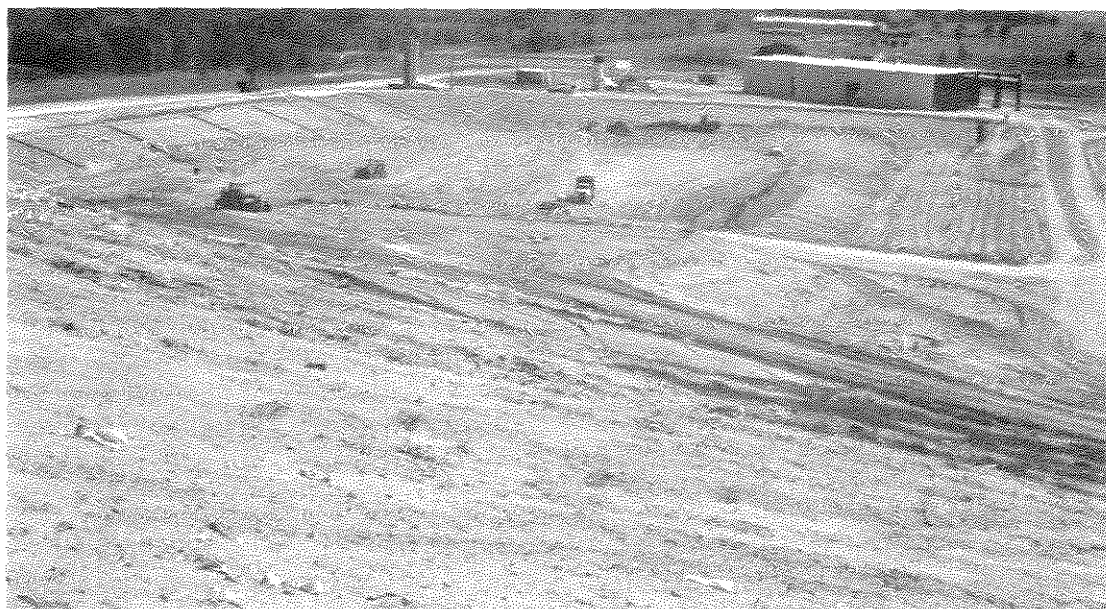
Figure 46. Newly opened cell at the Marion County landfill, showing plastic liner on left and background walls. The liner has been covered with sand on the other two walls for protection. Note the leachate collection pipes on the left and the 30,000 gallon holding tank in the left background. View to the south from the top of the recently finished, older cell, shown in Figure 45. Florida Geological Survey photograph, February 1989.
