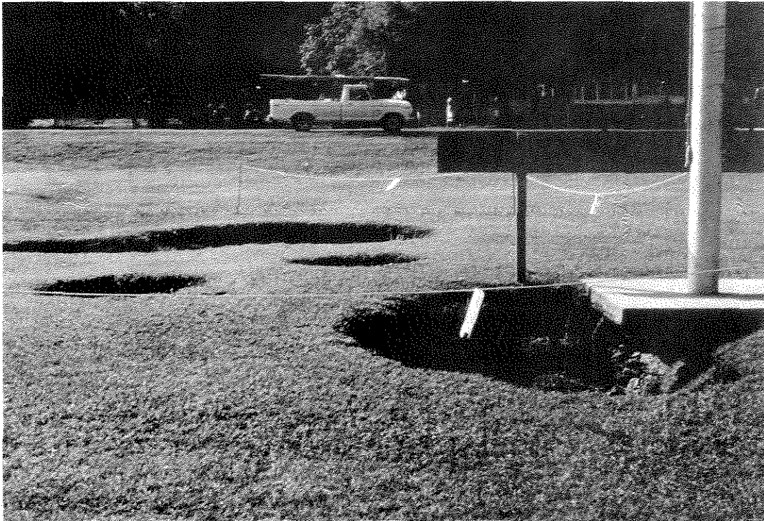
Figure 23. Sinkholes in City of Ocala formed during the flood of April 1982. Florida Geological Survey photograph.
