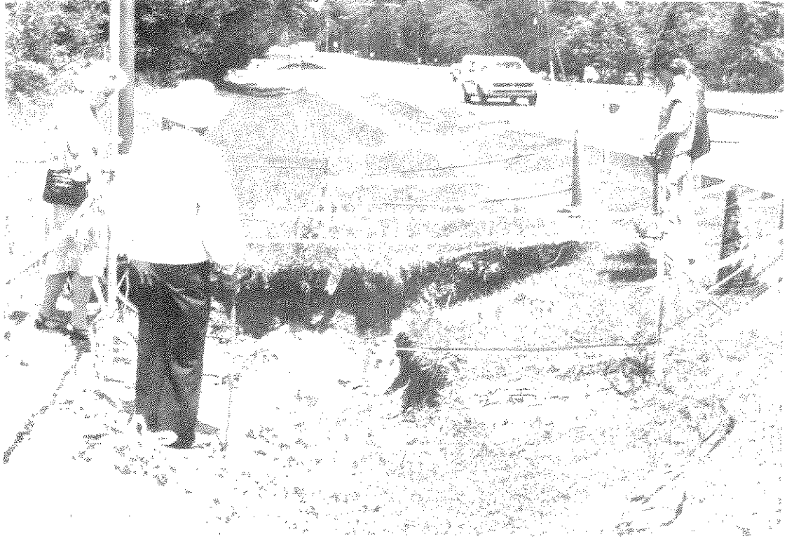
Figure 25. Sinkhole in City of Ocala formed during the flood of April 1982. Florida Geological Survey photograph.
